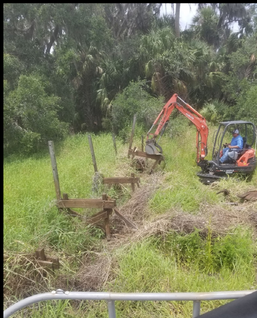
Mini-excavator pulling boardwalk pilings
