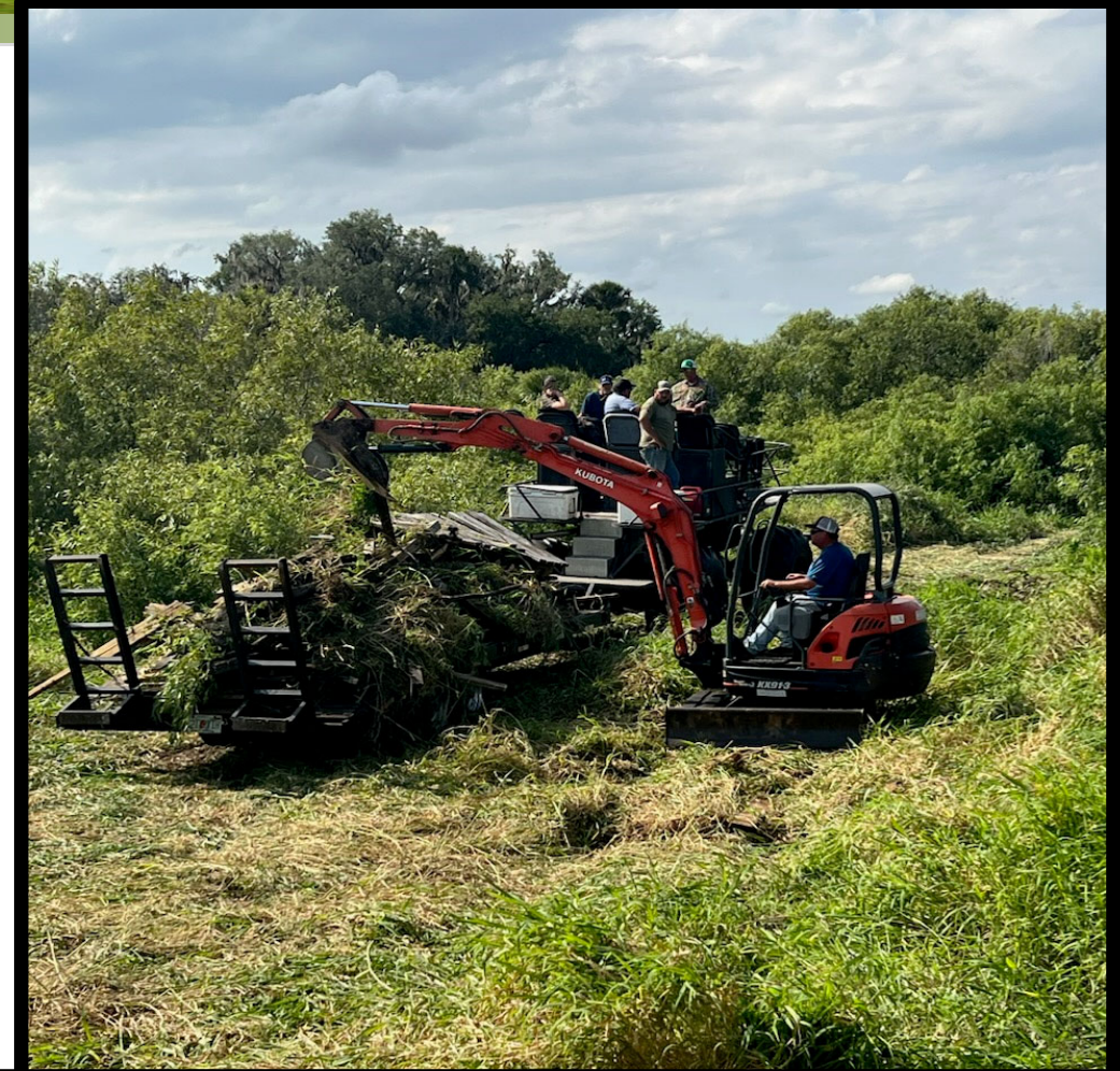
Mini-excavator loading trailer with boardwalk segments
