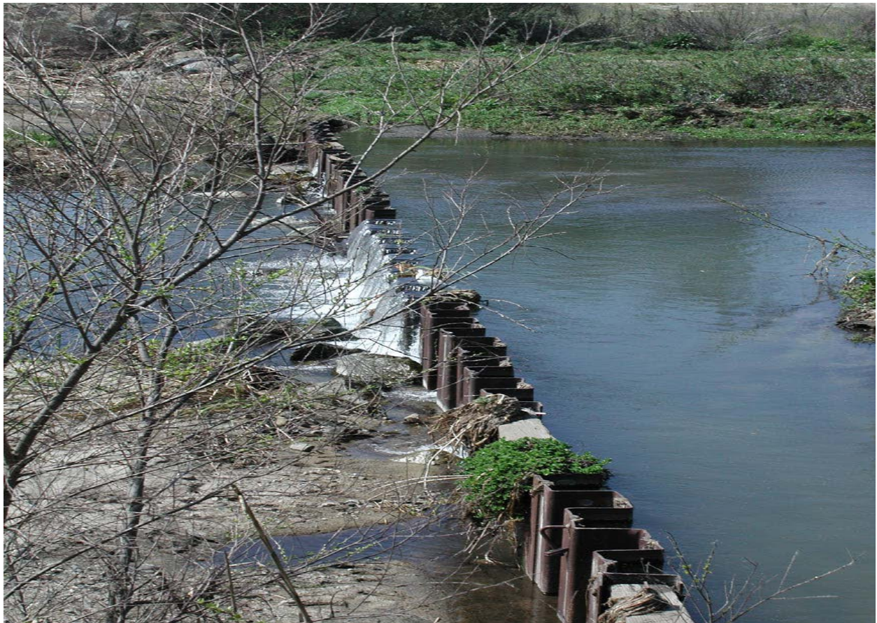
Figure E1. Sheet pile weir in the Santa Margarita River (from USBR, 2004)
