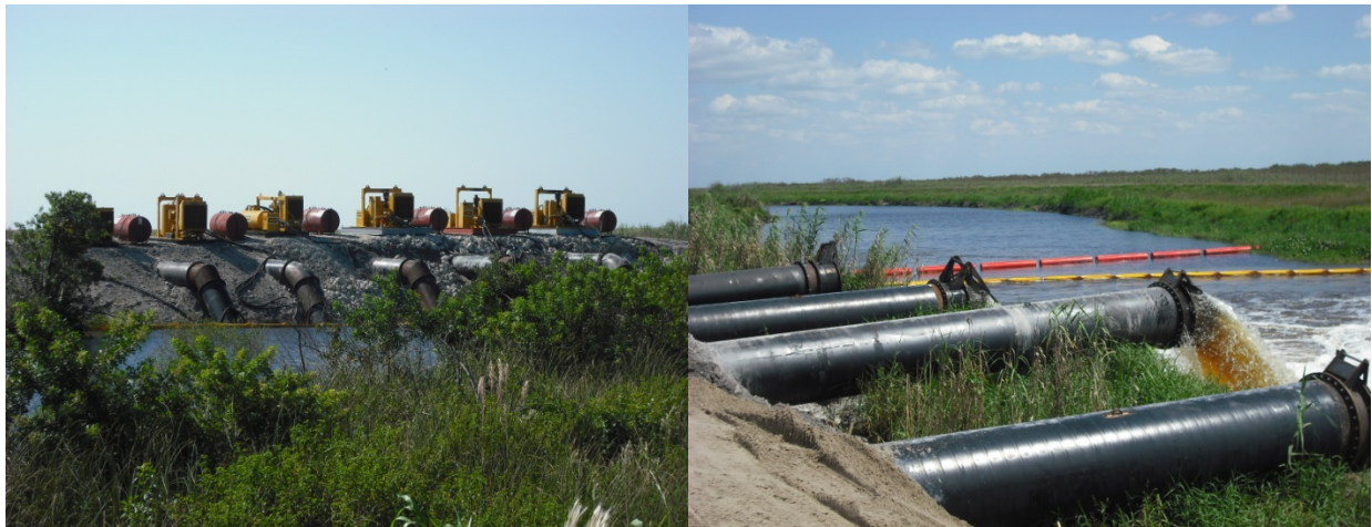
Figure G1. Temporary pump station at S-6 (head water at left, tail water at right)
