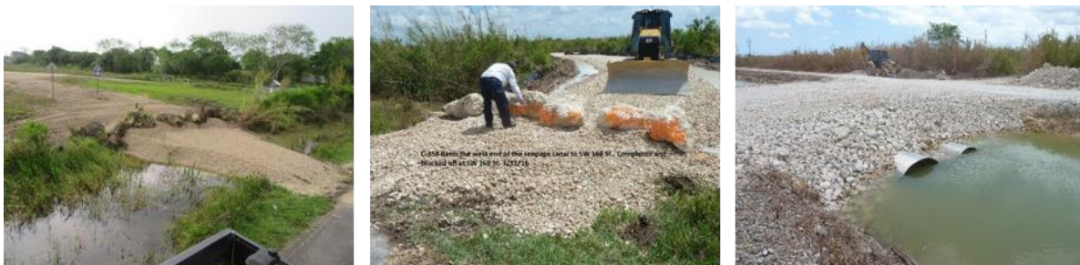
Figure 6. Las Palmas community mitigation (left to right): ditch plug on north side of Richmond Drive; berm connecting C-358 seepage collection canal berm to Richmond Drive; and culverted crossing of C-358 seepage collection canal.
