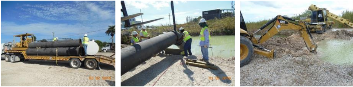
Figure 5. SFWMD transportation of power unit, pump, fuel tank, and pipe (left); connecting pipe (center); and removal of earthen plug (right).
