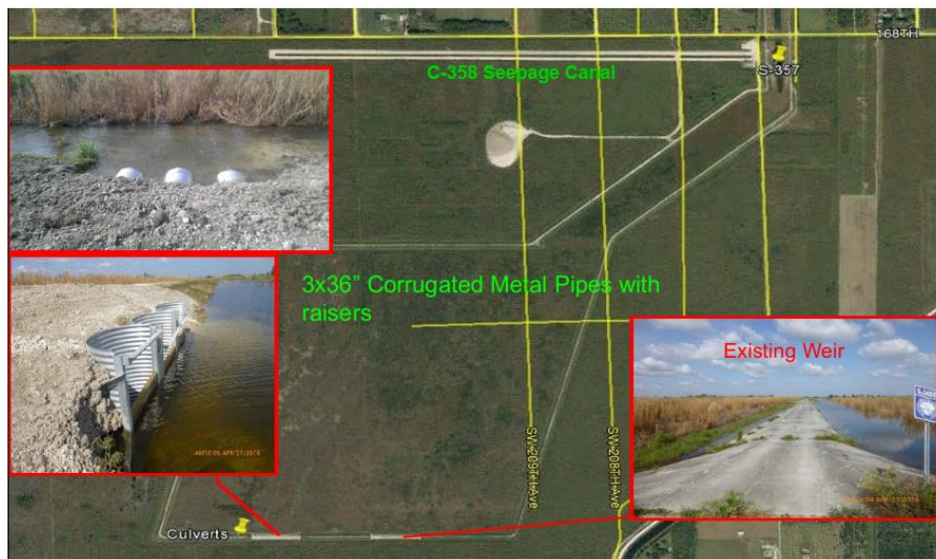
Figure 7. Temporary culverts at south end of the 8.5 Square Mile Area detention area.
