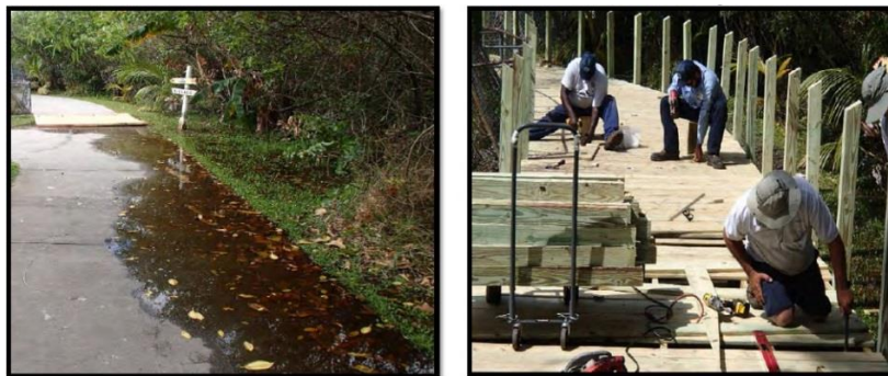
Figure 3. SFWMD installation of raised walkway with handrails at Everglades Safari Park.
