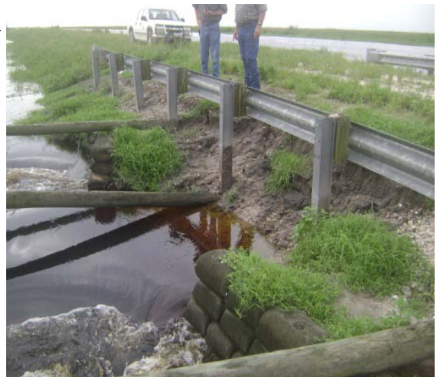
Eastern Culvert Headwall Failure
