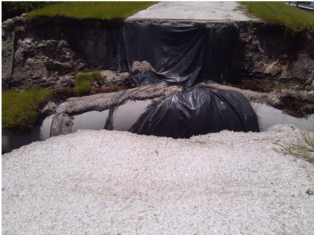
Preserve Area Drainage Culvert & Levee Road washout @ Lakeside Ranch STA
