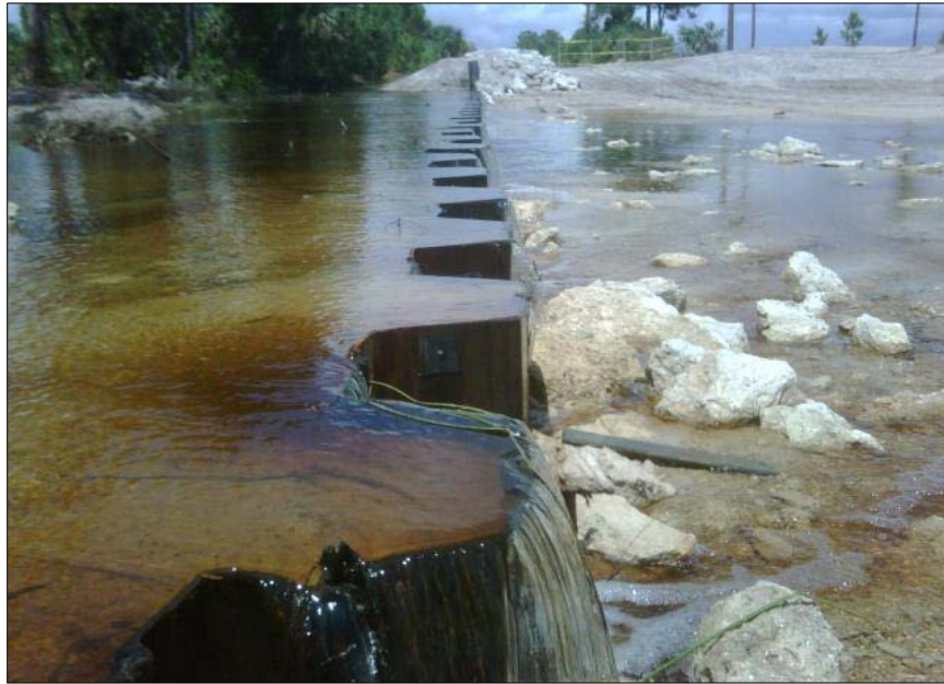
Interim repairs – Construction of 140 feet Overflow Weir
