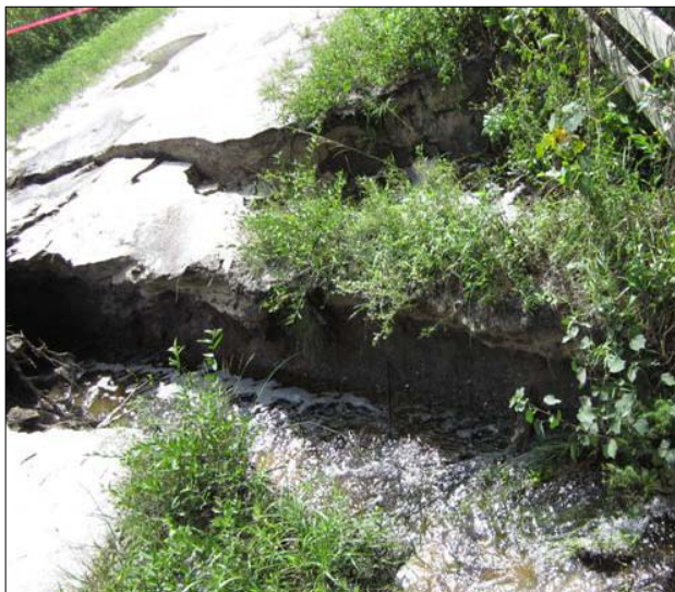
Roadway Collapse resulting from erosion
