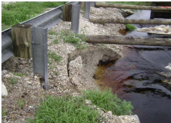
Center Culvert Headwall Failure
