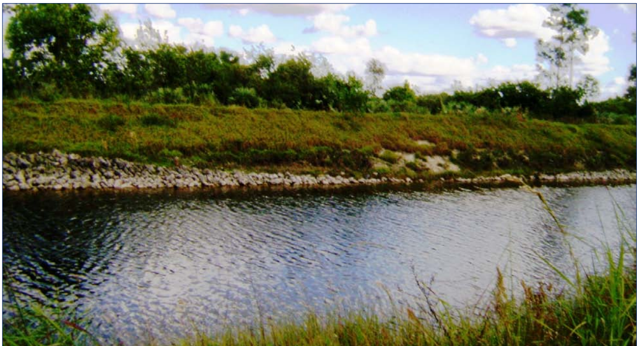
Failed section of rubble riprap
