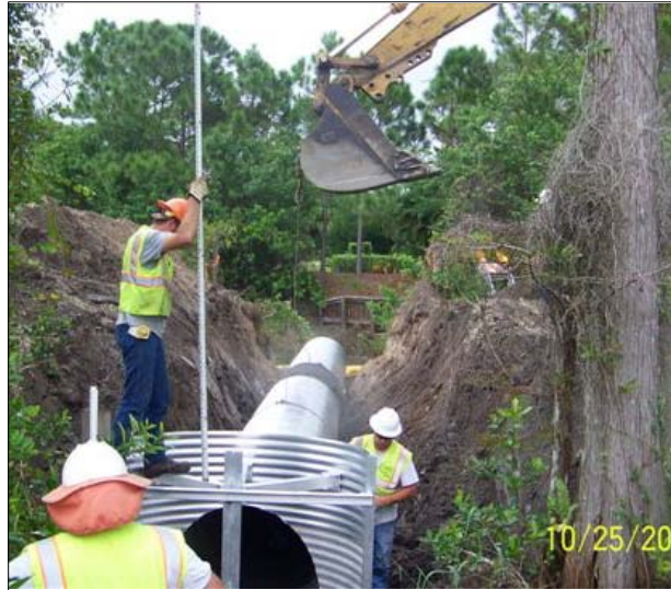
Installation of new Culvert Pipe by SFWMD Okeechobee Field Station Staff
