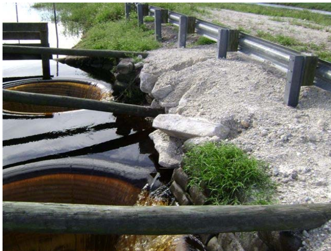
Temporary Repairs - Eastern Culvert Headwall
