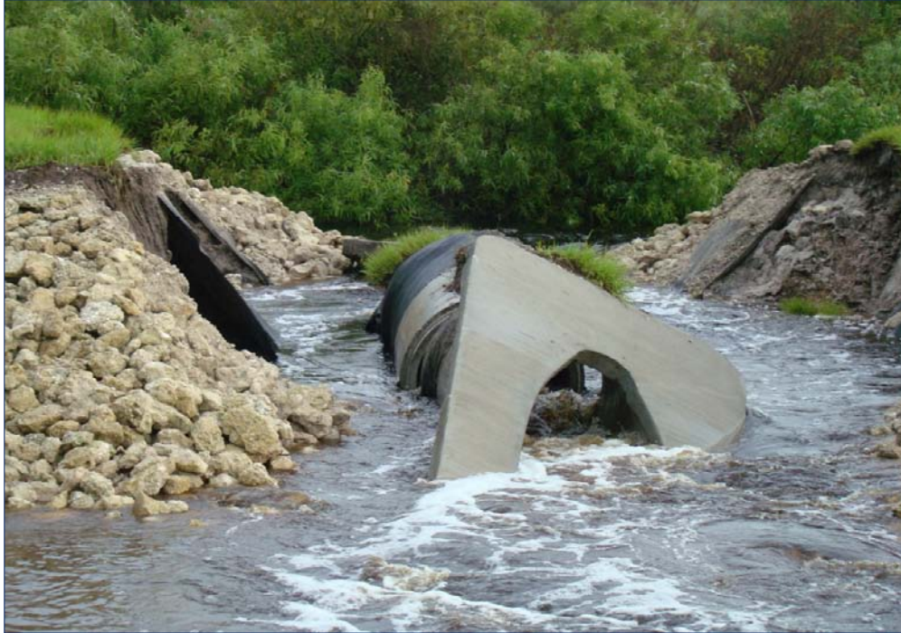
Preserve Area Drainage Culvert washout @ Lakeside Ranch STA
