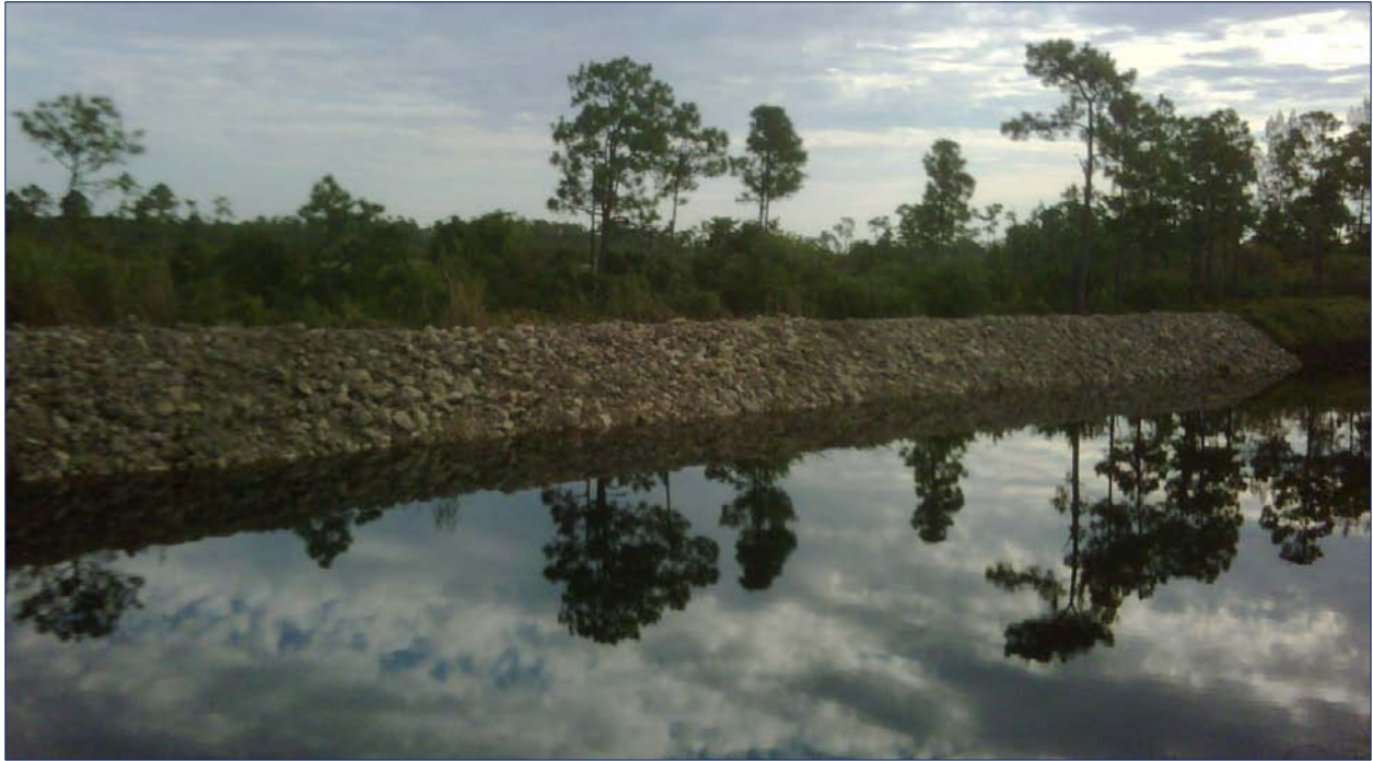
Typical Repair of ITID Berm Embankment
