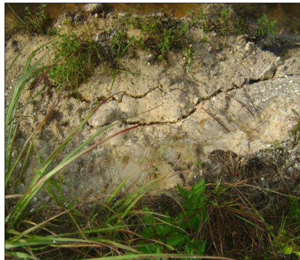
Berm Slope Failures, longitudinal cracks and boils due to high water levels
