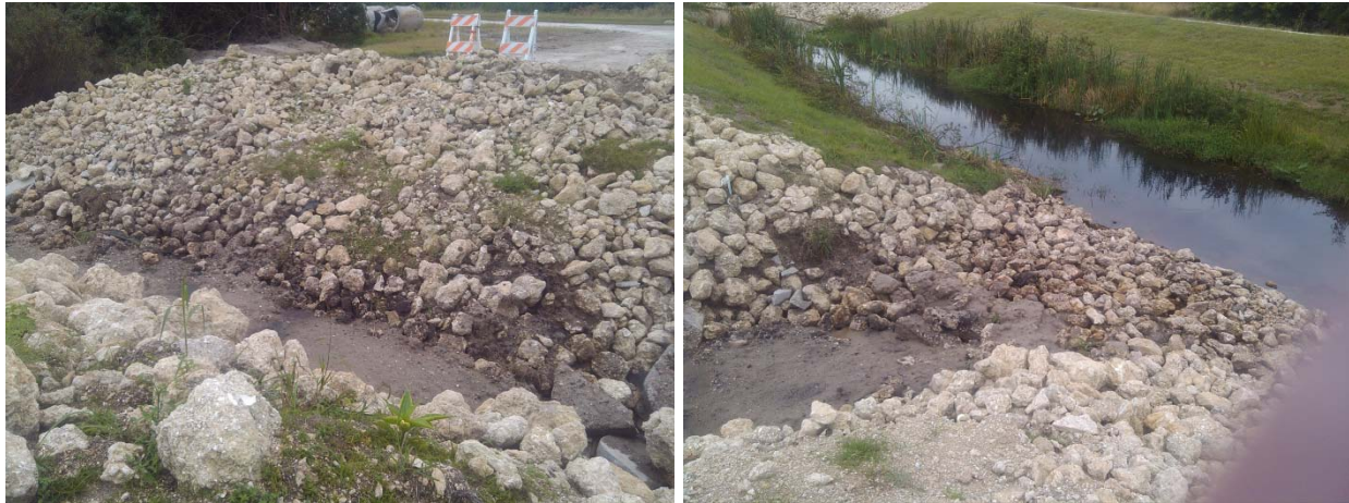
Temporary repairs @ Washed-out culvert location at Lakeside Ranch STA
