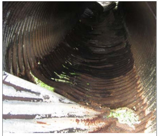
Damaged Culvert
