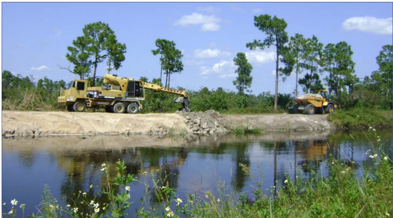
Repair of ITID Berm Embankment
