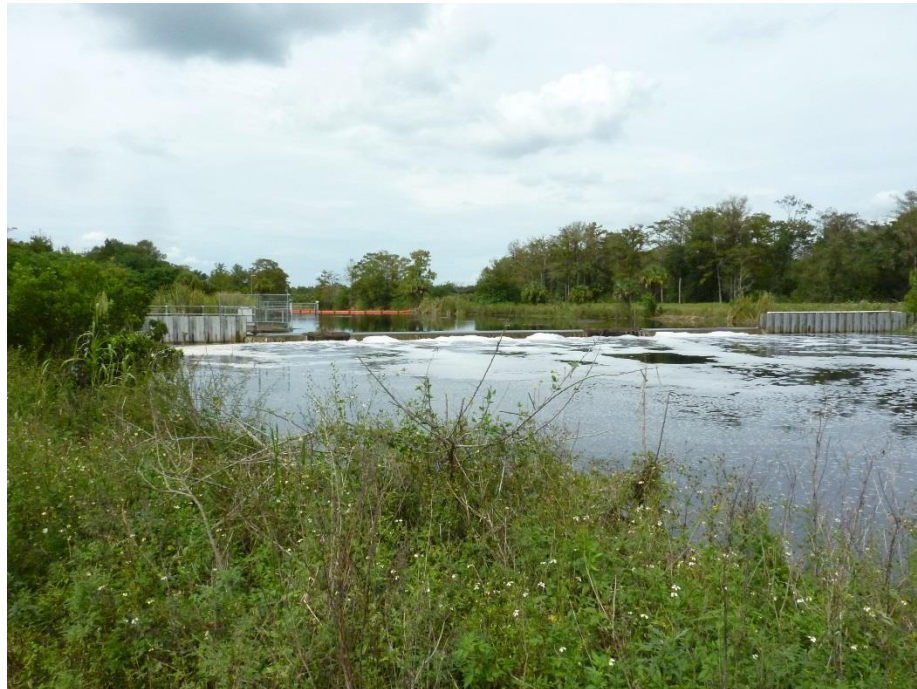
Figure 19: WWEIR Structure (Looking North and Upstream)
