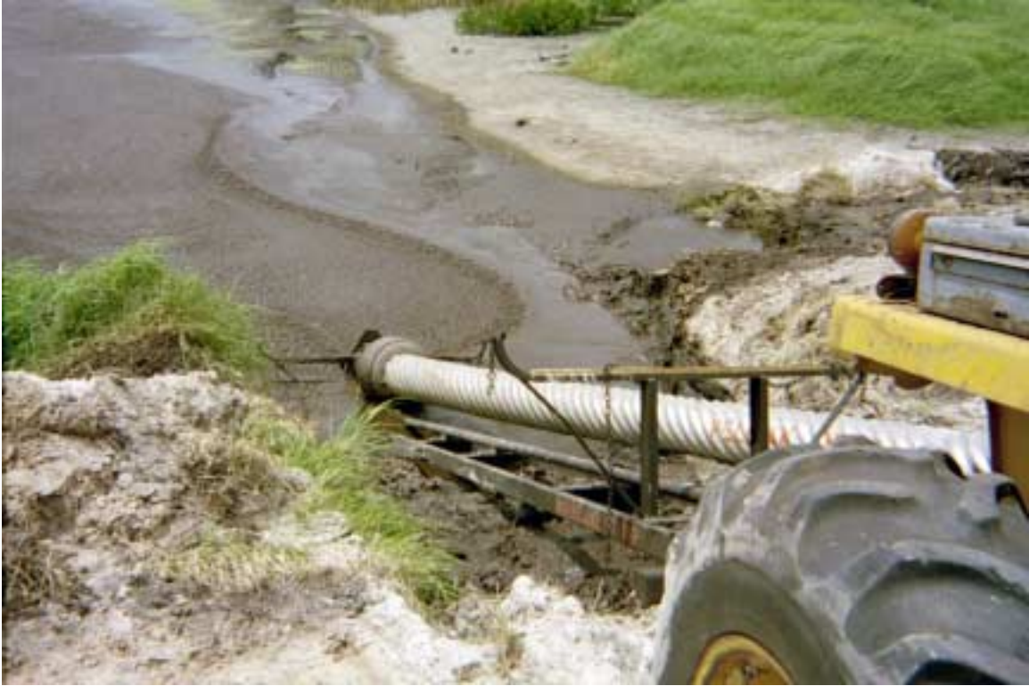
Figure 6. Pumping into Pond 1
