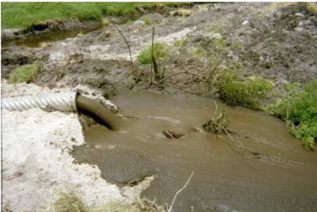
Figure 7. Discharge of pump into Pond 1
