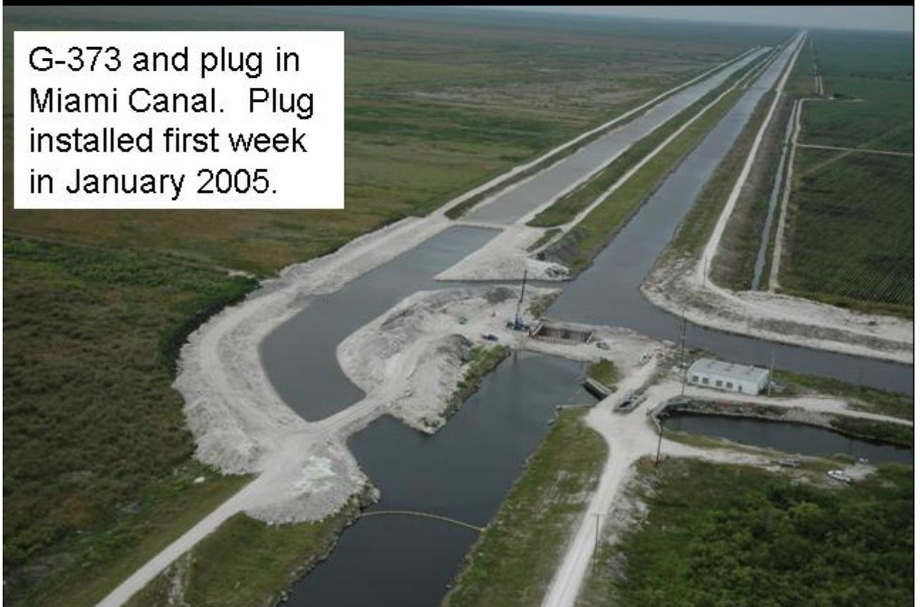
G-373 and plug in Miami Canal. Plug installed first week in January 2005.
