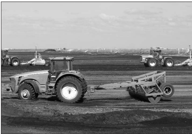
Enhancement work in Stormwater Treatment Area 1 West.
