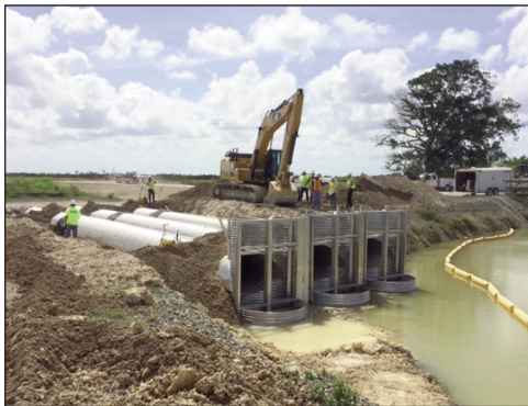
Crews install a canal connection that will deliver freshwater to Taylor Slough and Florida Bay.
