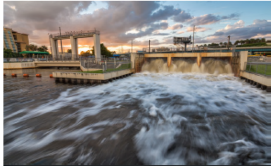
S-26 Pumping Station
