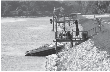
Permitting for some right of way uses is required, and structures must be built according to specifications.
