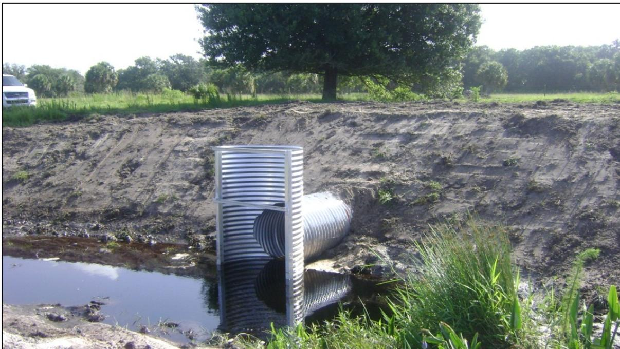
**Figure 10a.** Corrugated Metal Pipe with a Flash-Board Riser (Flash Board Fully Open)
