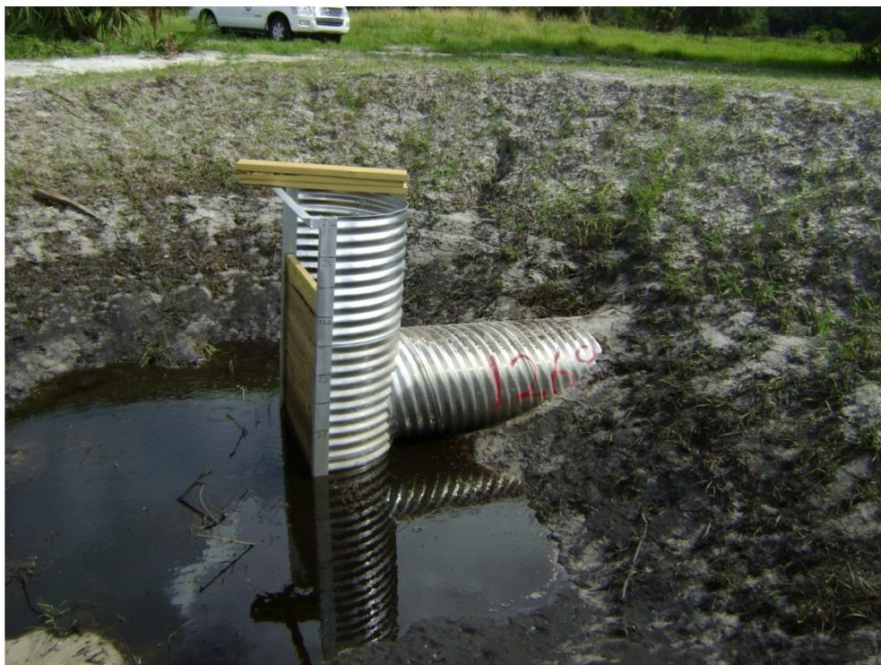
**Figure 10c.** Corrugated Metal Pipe with a Flash-Board Riser (Flash-Board Partially Closed)
