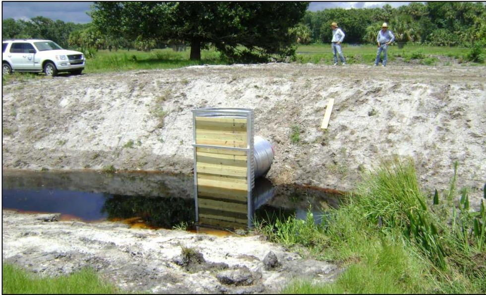
**Figure 10b.** Corrugated Metal Pipe with a Flash-Board Riser (Flash-Board Fully closed to the Top of the Riser)
