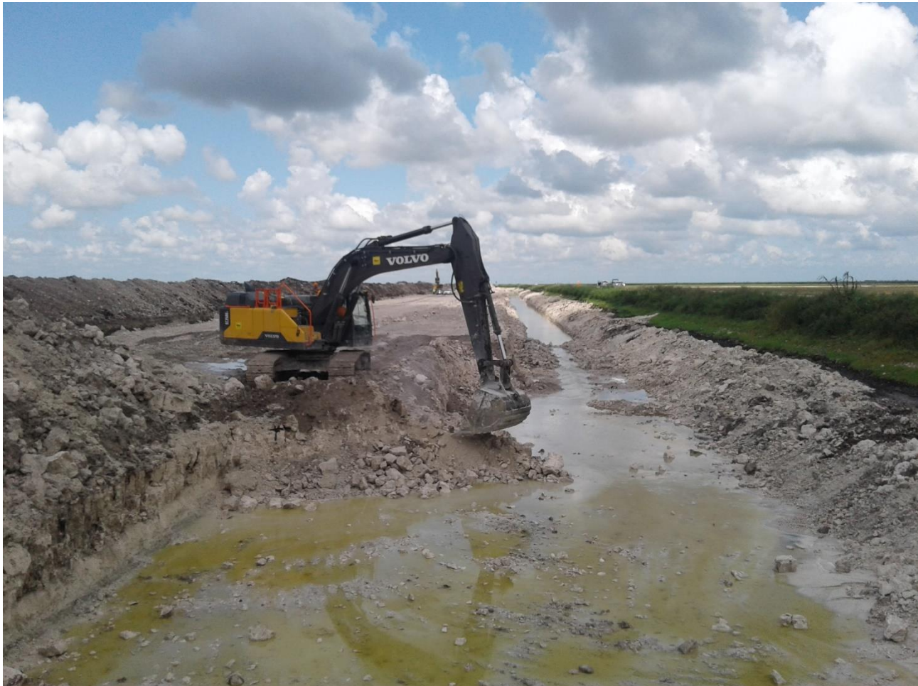
G-341 Related Conveyance Improvements – Bolles Canal Segment 3 construction (July 2018)
