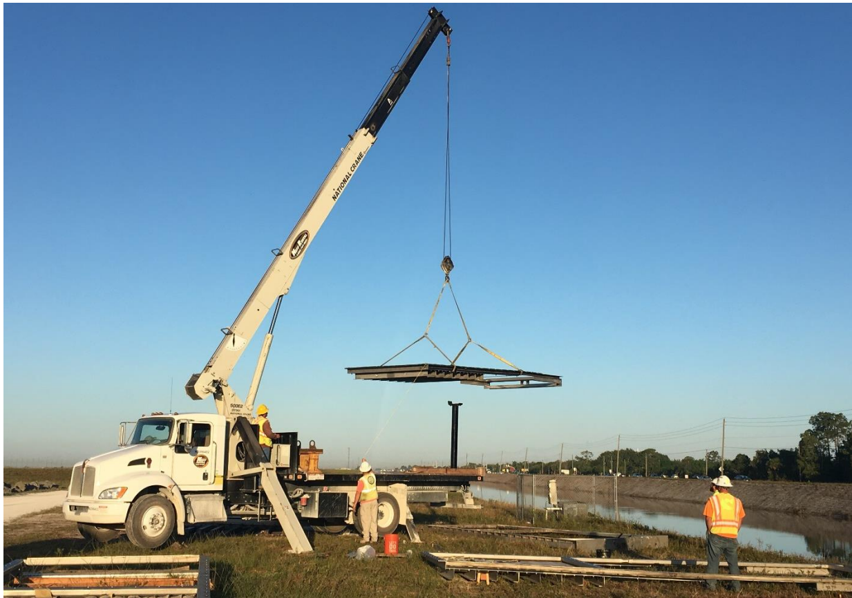
Slide Gate Repairs in STA-1E, Palm Beach County – March 2017
