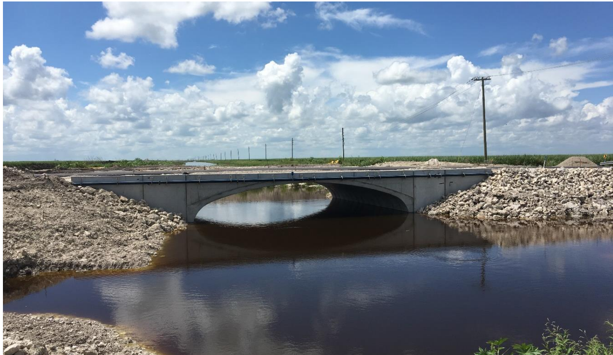
Duda Road Bridge in Palm Beach County – September 2016
