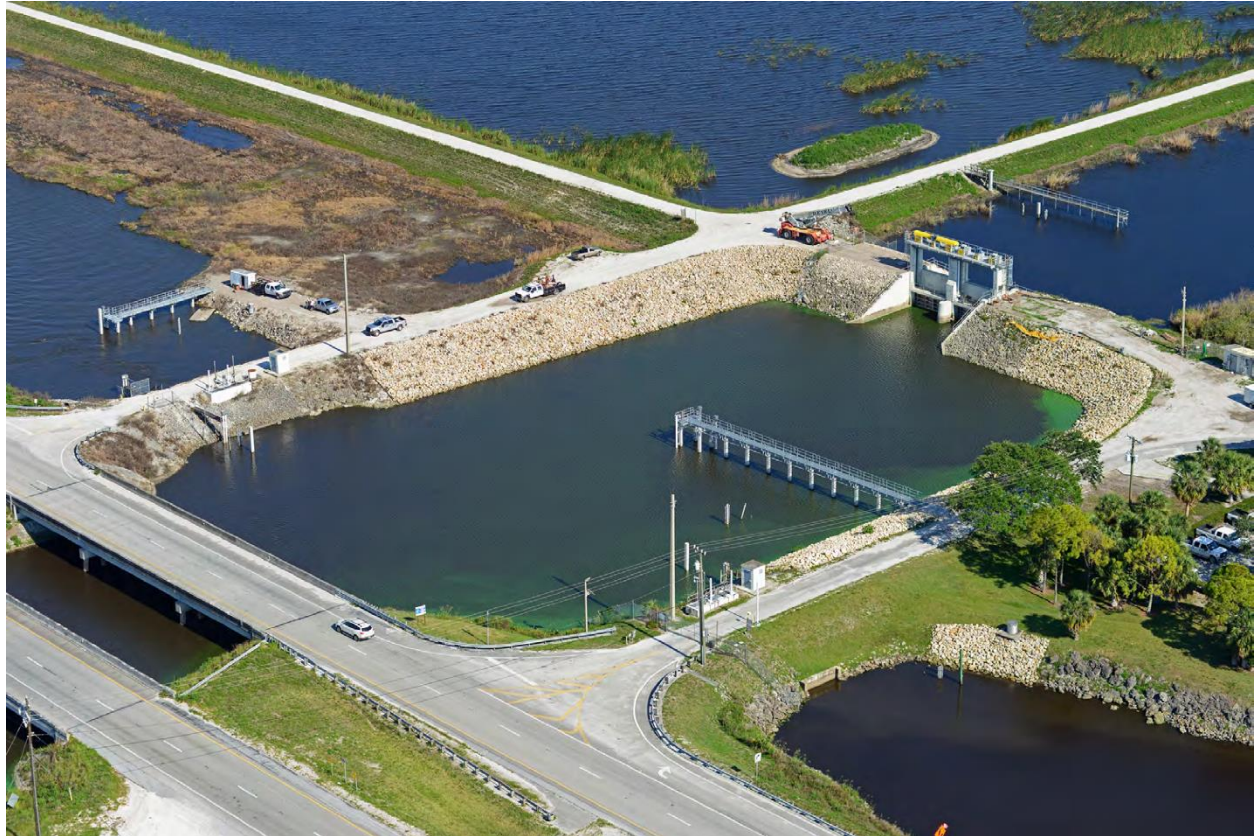
S-5AS Modifications (looking southeast) – May 2016
