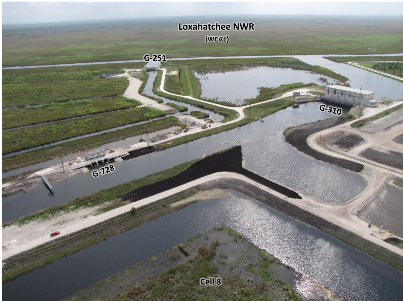
STA-1W Expansion #1: Discharge canal plug isolating G-251. Southeast view over Cell 8 facing southeast.
