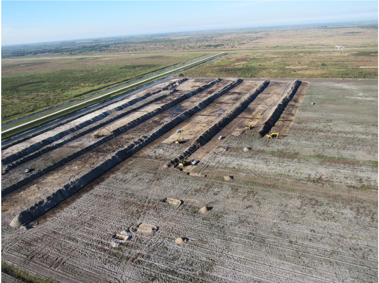
STA-5/6 Earthwork: SFWMD Field Operations regrading and stockpiling excess material in Cell 3A for hauling to C-139 FEB site. View facing southwest.
