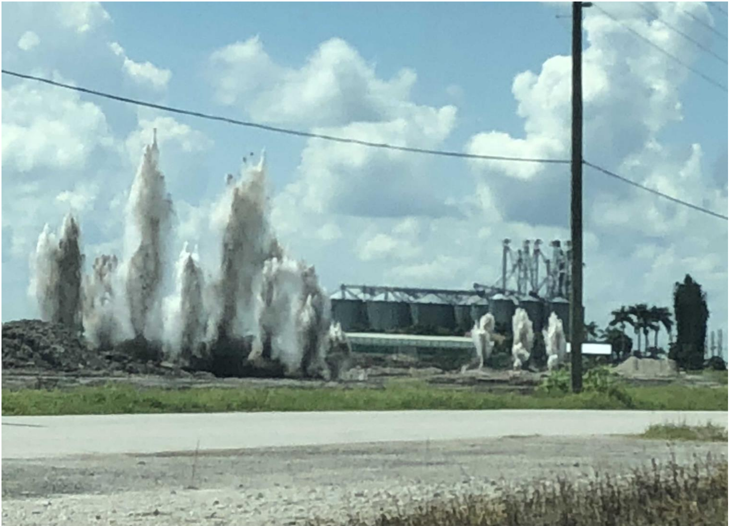
STA-1 W Expansion#1: Blasting of the collection canal in the north west corner of Cell 6(September 2018)
