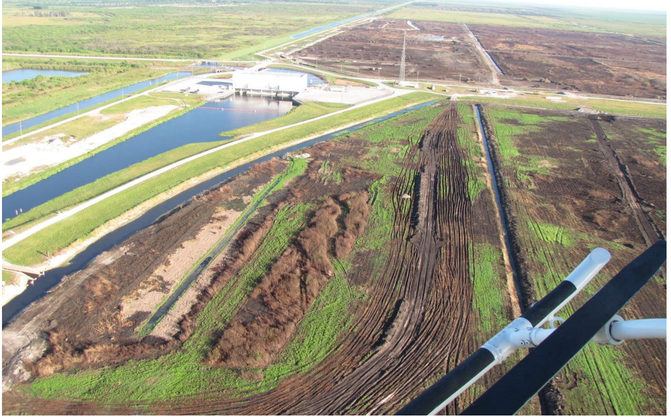
STA5/6 Internal Improvements: Earth moving preparations in Cell 2A and Cell 3A.
