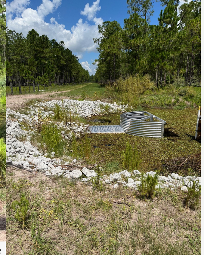
Image of 60" riser culvert replacement in the Big Bend Swamp
