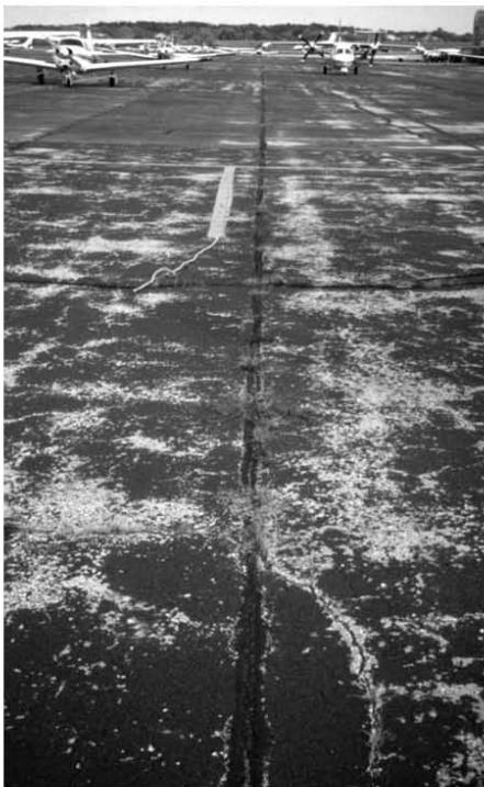
◀ Joint sealant needs replacement at several locations. Follow with new surface treatment on apron.
