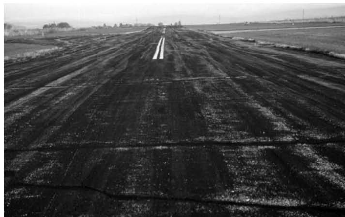
▼ Worn sealcoat needs new surface treatment.
