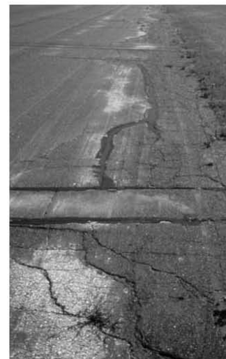
▼ Repair broken pavement and apply overlay.
