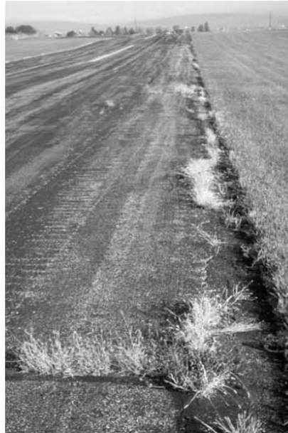
◀ More than 25% of crack sealant needs replacement. Minor settlement over cracking.
