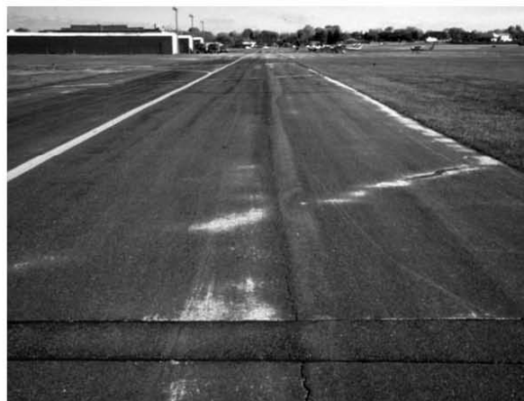
▼ Worn sealcoat needs new surface treatment.
