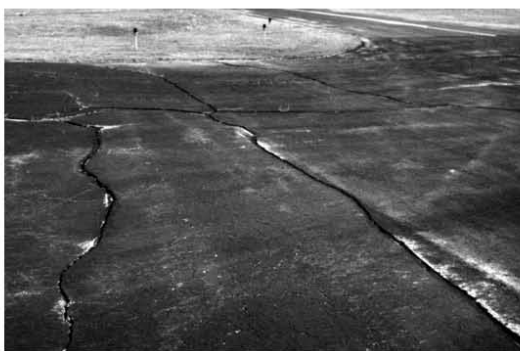
◀ More than 25% of crack sealant needs replacement. Minor settlement over cracking.
