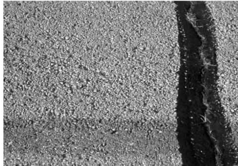
◀ Moderate raveling. Joint needs sealing.
