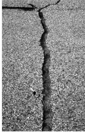
▲ Wide cracks with no sealant.
