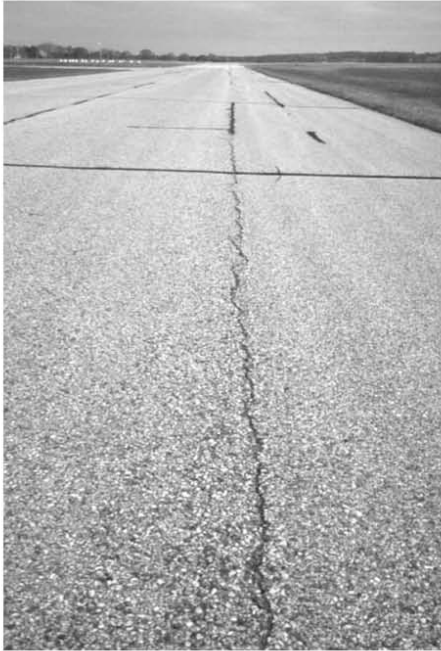
◀ Moderate raveling. Joint needs sealing.
