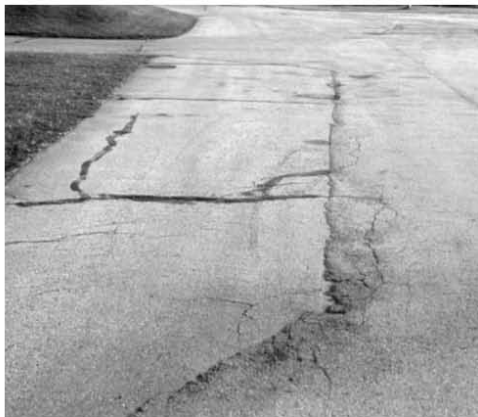
▼ Overlay repair with edge raveling and cracks.
