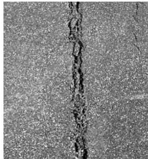
▲ Wide cracks with no sealant.
