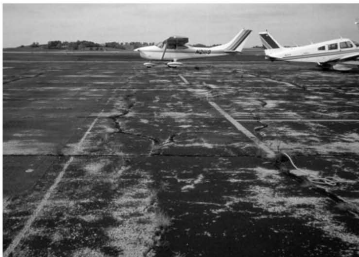
▼ Sealant repair needed on more than 25% of cracks.
