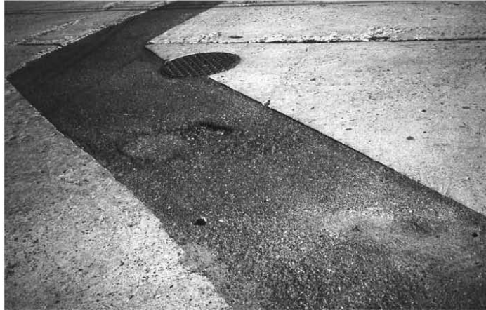
▲ Typical repair of utility excavation. Patch in good condition.
