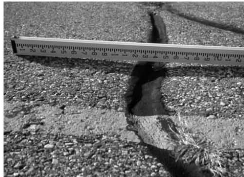
◀ Edge cracking at several locations.
