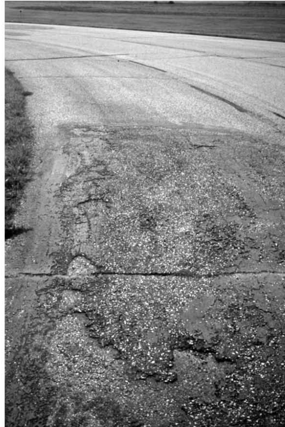
▶ Patched area in poor condition.
