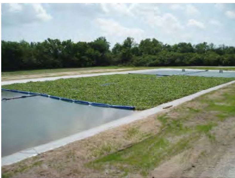
Figure 4-8: Hybrid Wetland Treatment Technology 13
