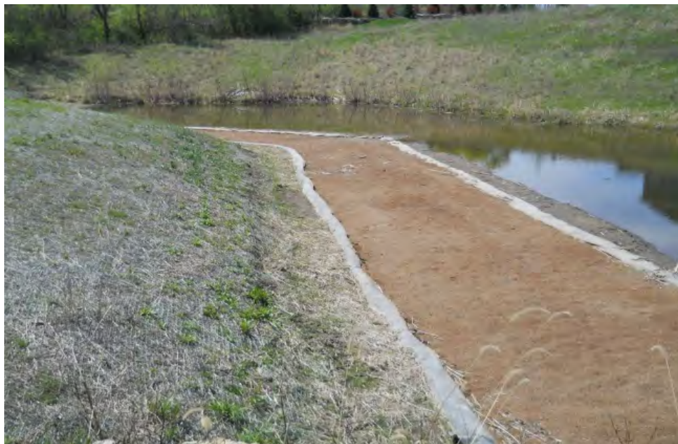
Figure 4-11: Iron Enhanced Sands Filtration Example 17
