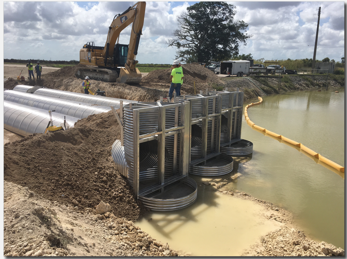
Crews install a canal connection that will deliver freshwater to Taylor Slough and Florida Bay.
