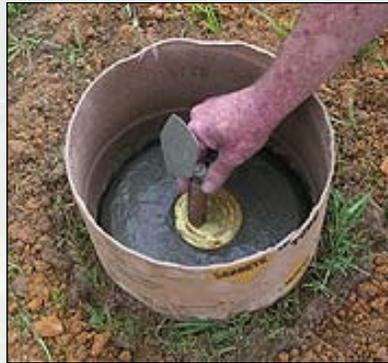
Bronze or Brass disks set in poured-in-place concrete, or existing structure with a deep foundation.
