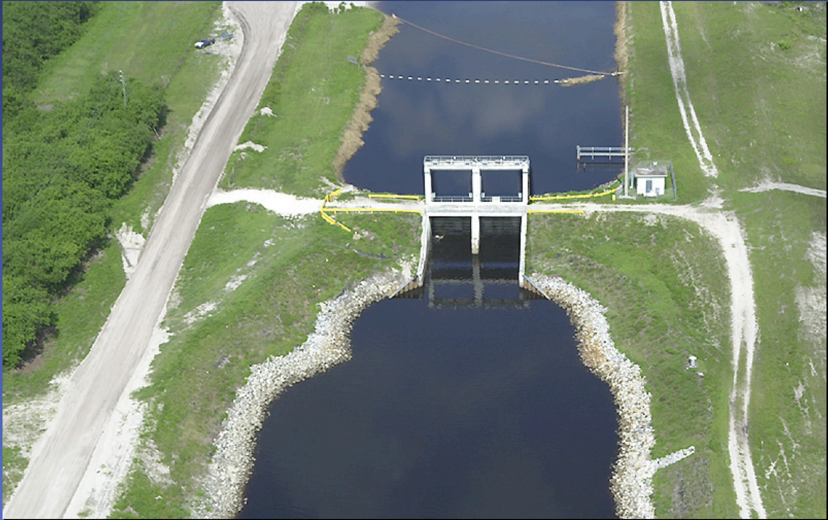
C-23 Canal Control Structure S-97
