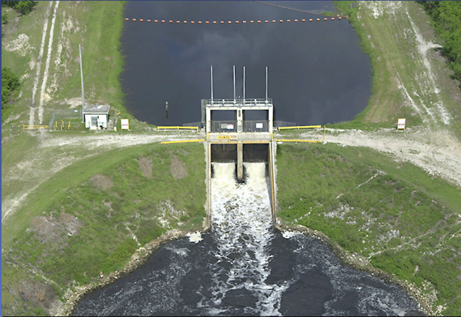
C-24 Canal Control Structure S-49
