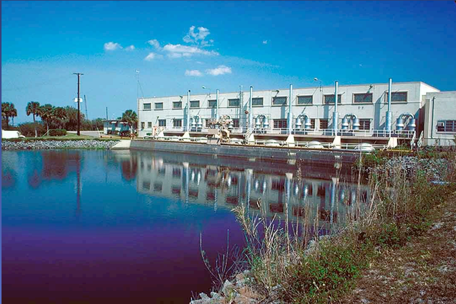
Pump Station 5A (WCA-1) in Palm Beach County
