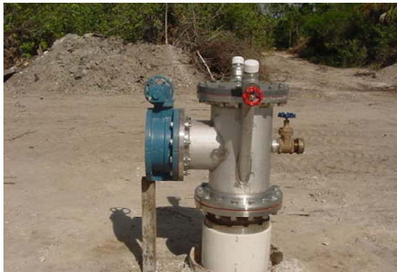
Aquifer Storage and Recovery Well
