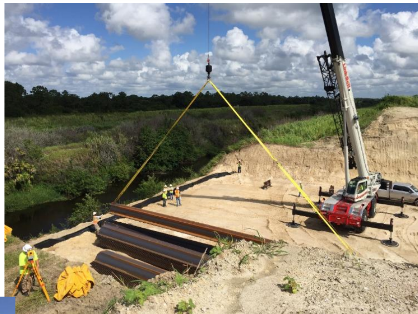
Installation of Sheet Pile at PS 476
