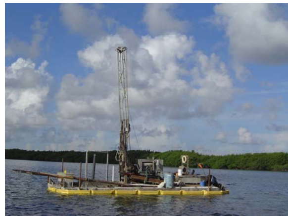
Installation of Saltwater Monitoring Wells
