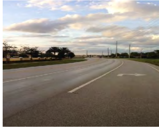
Facing north along Canoe Creek Road (Photo Taken on January 9, 2014)
