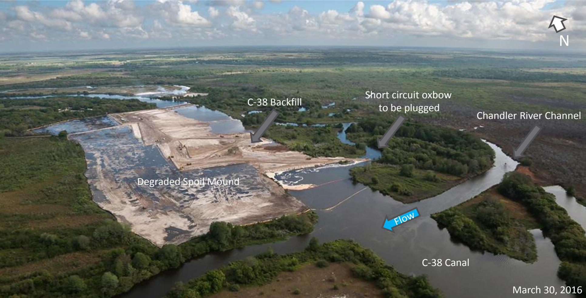
Looking north at Reach 3 restoration area. Contractors are constructing a plug across the short circuit oxbow to divert flows through the main Chandler River Channel.
