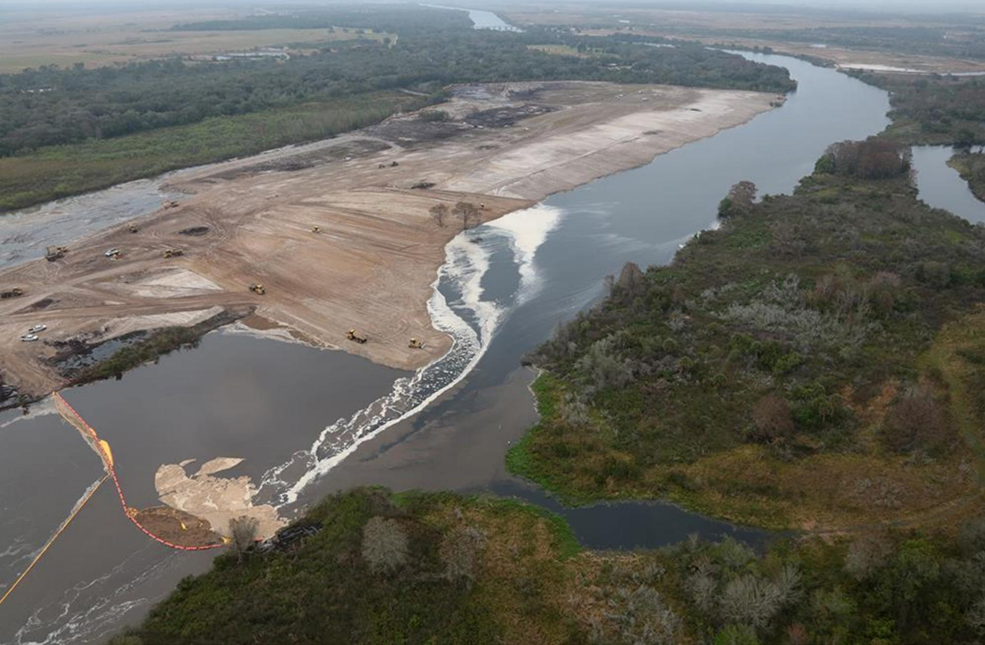
Kissimmee River Reach 3 restoration area looking northwest. Contractors are pushing spoil across the C-38 canal to create the initial plug of Reach 3 backfill.
