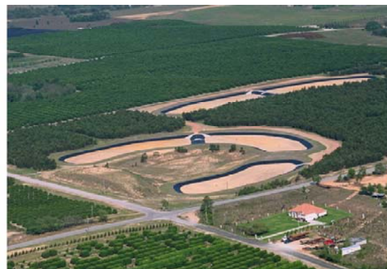
Rapid Infiltration Basin
