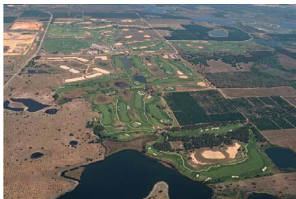
Golf Course and Rapid Infiltration Basins
