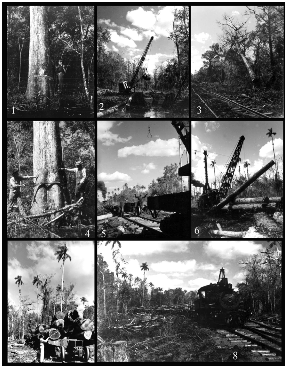
Tram Logging: 1) scouting parties girdle virgin cypress up to a year before logging to allow the stored water to drain out; 2) tram roads are created with a diesel dragline that dredges adjacent soil and muck to build up the road bed; 3) narrow gauge rails are laid on the tram roads, called “dummylines”; 4) logging teams fell the trees; 5) rail cars forming a train; 6) steam skidder loading cypress logs; 7) measuring the diameter of felled logs; and 8) hauling the trees to a local mill which, at its peak, was producing 100,000 board feet of lumber a day.
