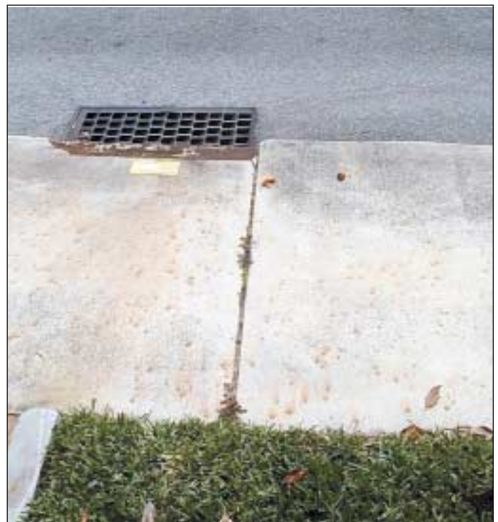
Figure 3. Poor fertilization technique wastes fertilizer, causes unsightly stains, and pollutes our waterbodies. Note the trail of stains on this sidewalk.
