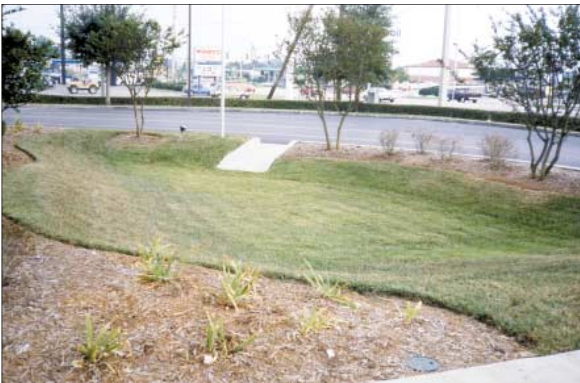
Figure 2. Grassy stormwater retention areas can add dimension to a lawn and protect our environment.
