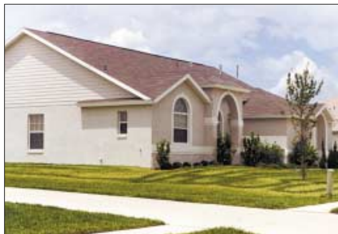
Figure 19. Streaking on a lawn caused by poor application techniques.
