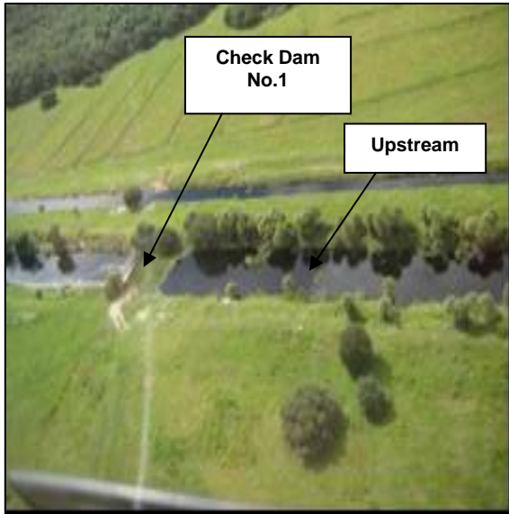
Figure 8. PL-566 Check Dam No.1 Structure on FEC (Looking W)
