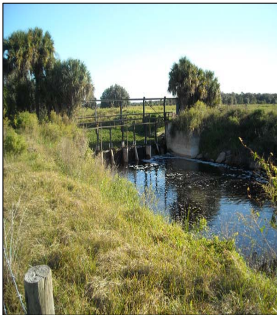
Figure 10. A View of Check Dam No.1 Structure from Downstream
