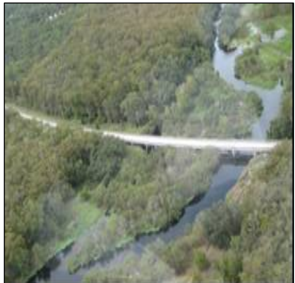
Figure 15. FEC – CR 731 Intersection (Looking South)
