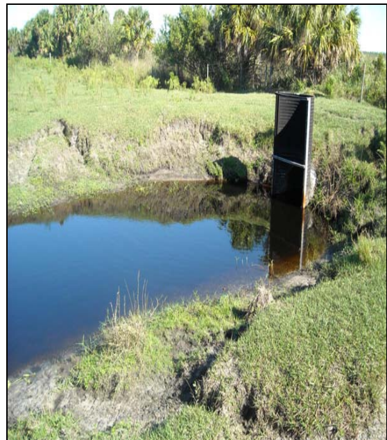
Figure 11. Culvert Located at the Upstream of Check Dam No1 (27.27513 N, 81.47126 W)
