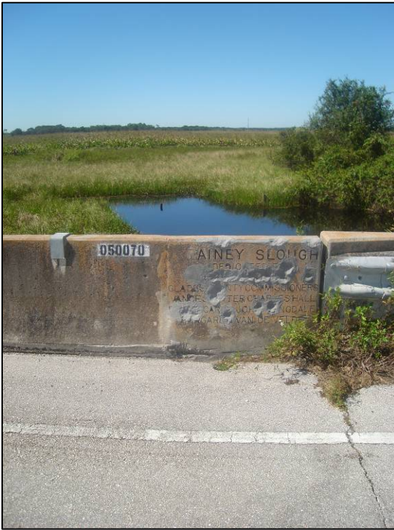
Figure 70. Rainey Slough, View to the West
