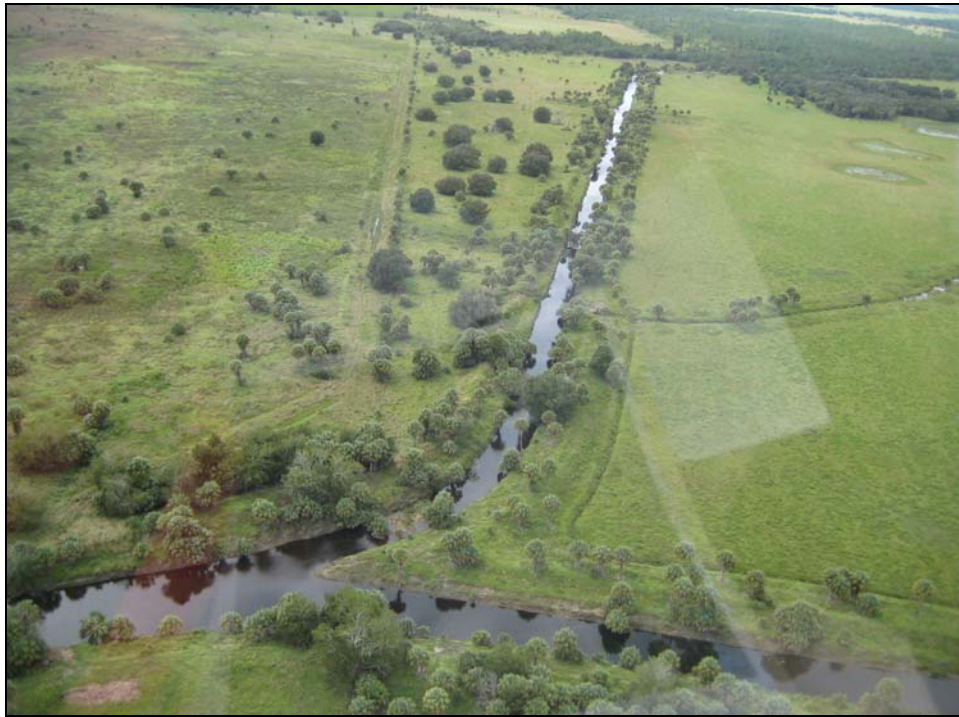
Figure 80. An Aerial View of the Upper Reaches of FEC, North Lateral to Left
