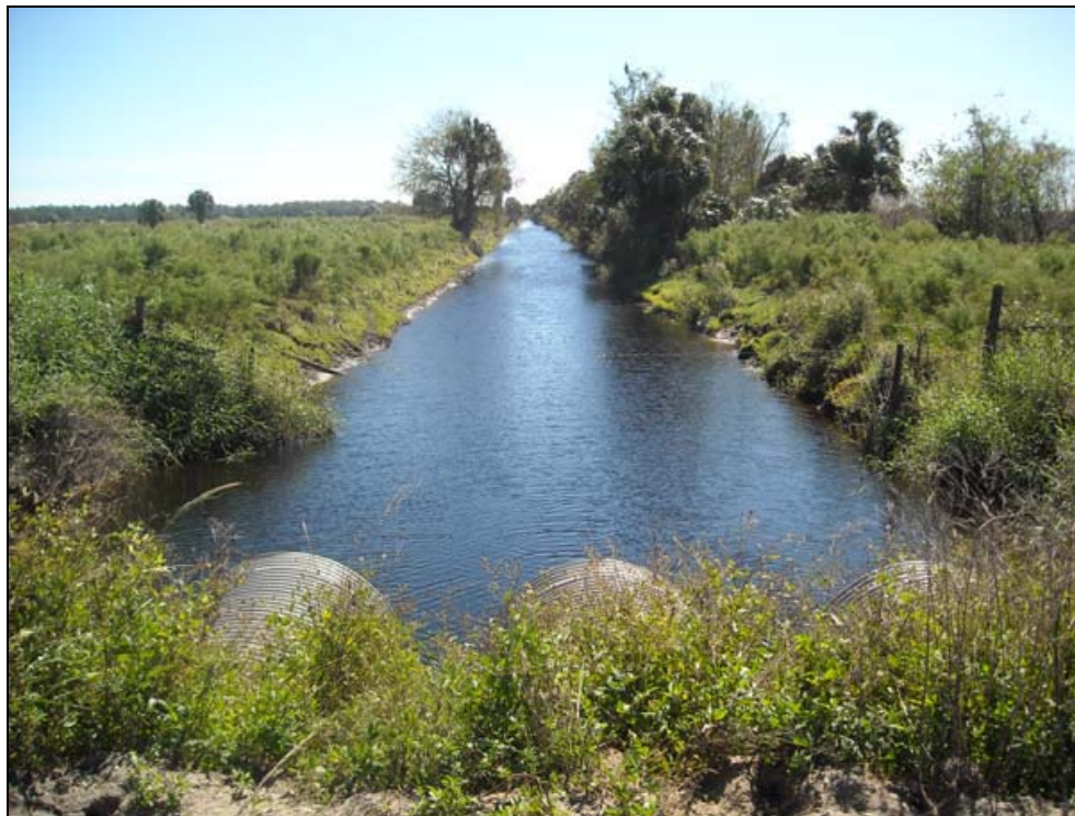
Figure 81. View of Channelized Portion of Fisheating Creek, Looking N
