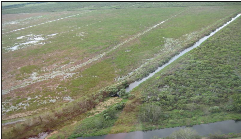
Figure 65. FEC South Intercept, Looking NW
