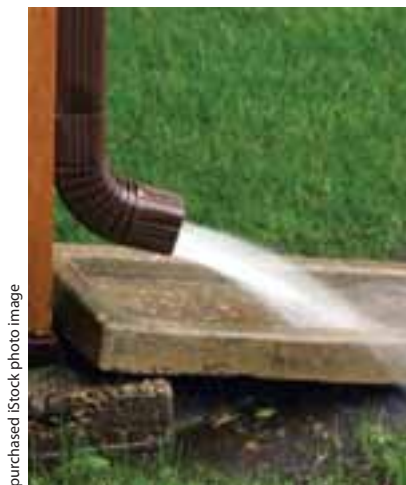
Downspout directed into the yard.
