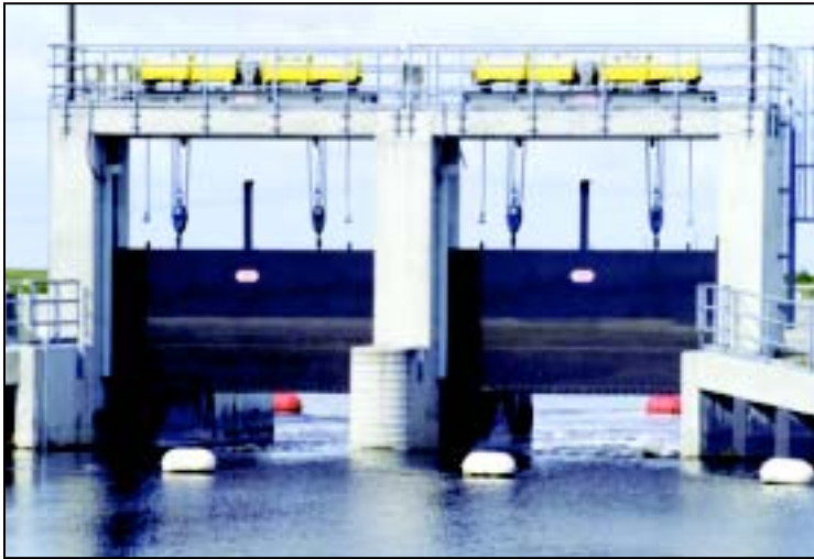
LARGE GATED STRUCTURES AND PUMPS, SUCH AS G-302 AT STA-1W, ARE USED TO MOVE WATER THROUGH THE STAS.
