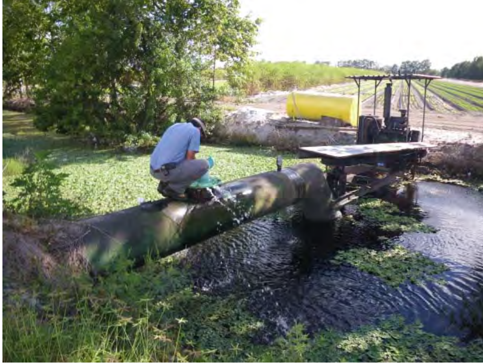
Figure 10. Pump calibration using propeller-type flow meter, elapsed time, pump speed and borrow ditch stage level
