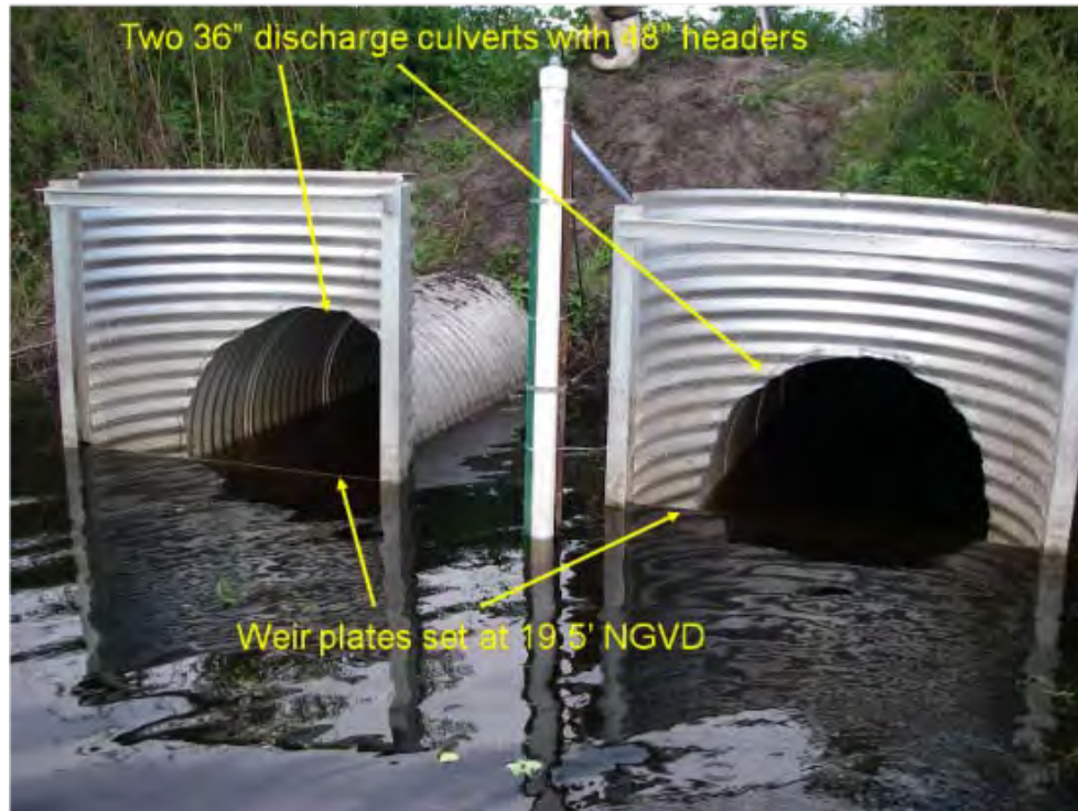
Figure 11. Water control structures and associated control elevation at the discharge site.
