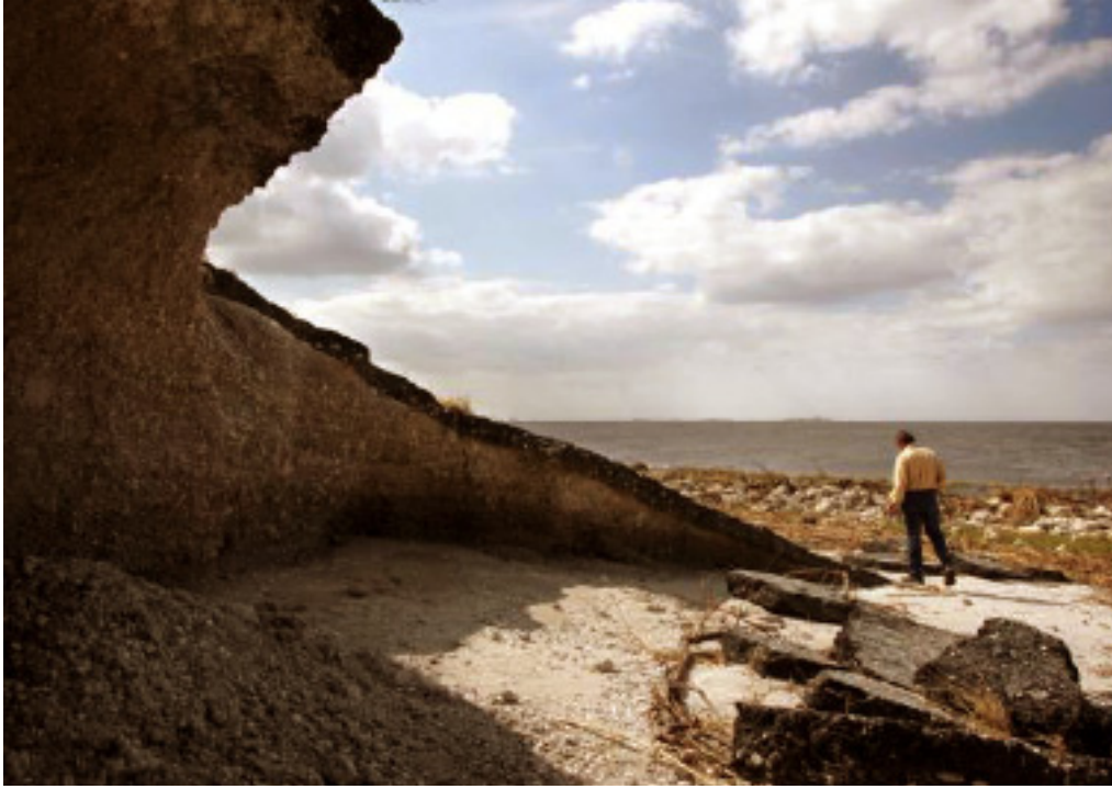
Figure 7. Wave erosion damage to the Herbert Hoover Dike of Lake Okeechobee from Hurricane Wilma (Bromwell et al., 2006).
