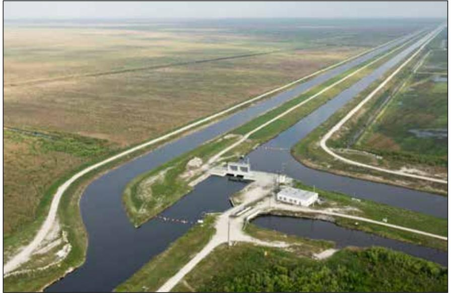
**The Miami Canal (bottom right) is one of two canals where conveyance improvements would be made to ensure the EAA Storage Reservoir works as intended.**
