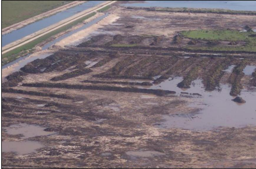
**Figure DBE-1.** Photo of substrate preparation during PSTA Cell construction. Organic soils were scraped from limerock, then removed or formed into berms that extend perpendicular to the dominant (north-to-south) flow direction.
