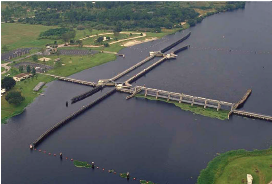
Structure S-79 on the Caloosahatchee River
