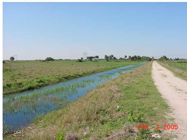
Photo 2.1 Typical Farming Ditch along dirt road in Bear Slough; ditch acts as a basin divide
