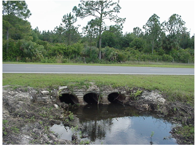
(Left) Photo 2.7 Citrus Grove Pumping Station located at northeastern boundary of Corkscrew Marsh (Right) Photo 2.8 Concrete tri-culverts conveying agricultural runoff into Corkscrew Marsh
