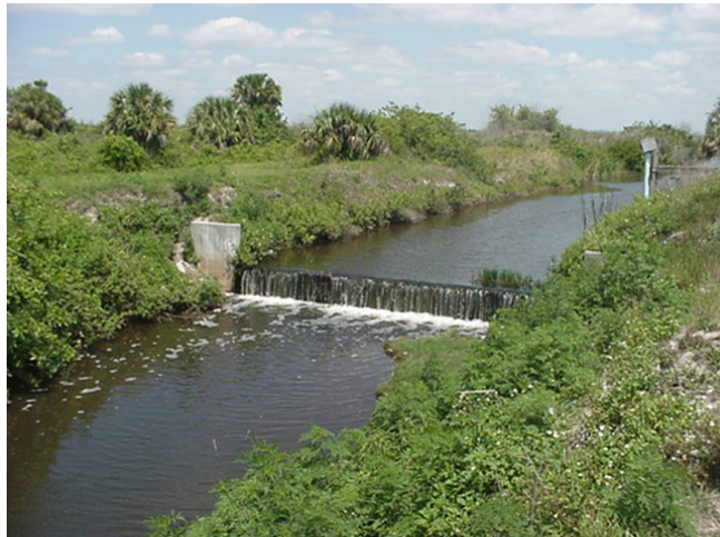
Photo 2. 6. Fixed crest concrete weir located at entrance into CREW management center.
