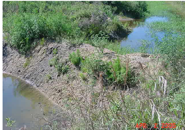
Photo 2.5 Typical Farm Berm in Canal, Camp Keais Sub-Basin
