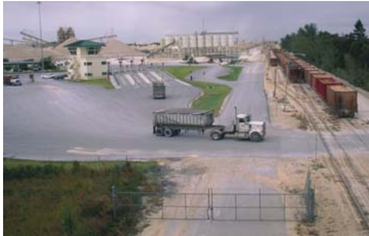
Substantial amounts of public and private infrastructure have been built within and around the Lake Belt Area
