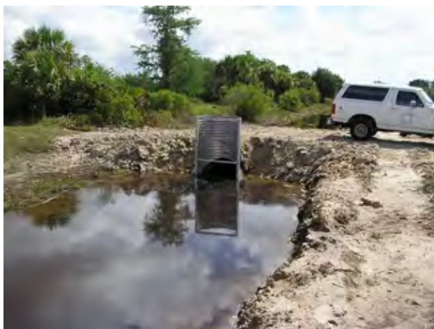
Culverts with risers for water management and with mud boards for sediment control
