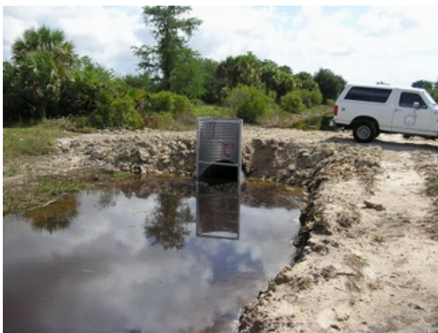
Culverts with risers for water management and with mud boards for sediment control
