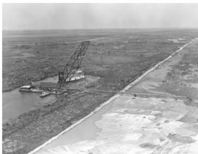
*The Kissimmee River was “channelized” to manage its water flow. Over the course of nine years (1962-1971), the meandering river was cut and dredged into a straight canal (C-38) with six water control structures. Two-thirds of the original floodplain was drained.*
