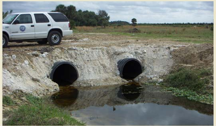
Culvert installation and stabilization
