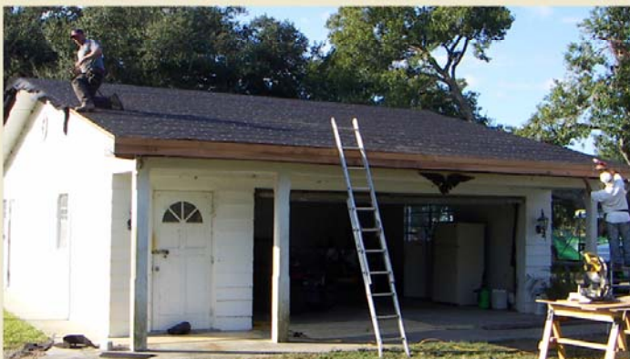
A new roof being installed on District property
