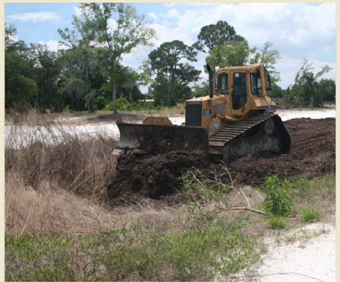
Plugging drainage ditches at River Runt
