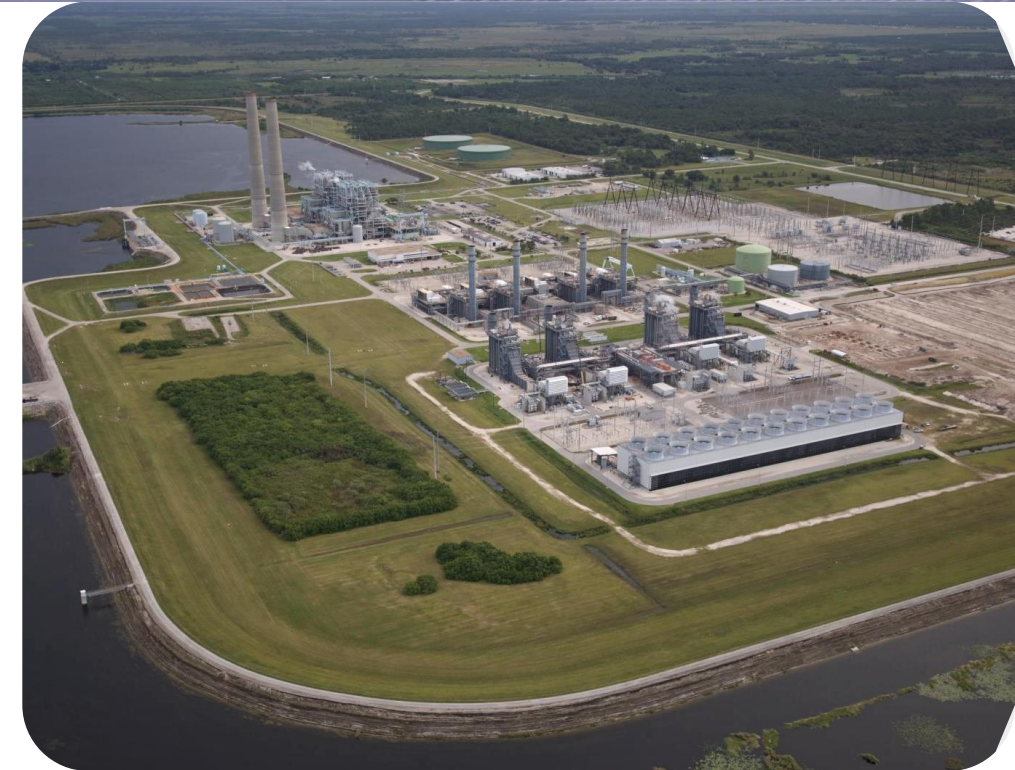
Martin Power Plant
