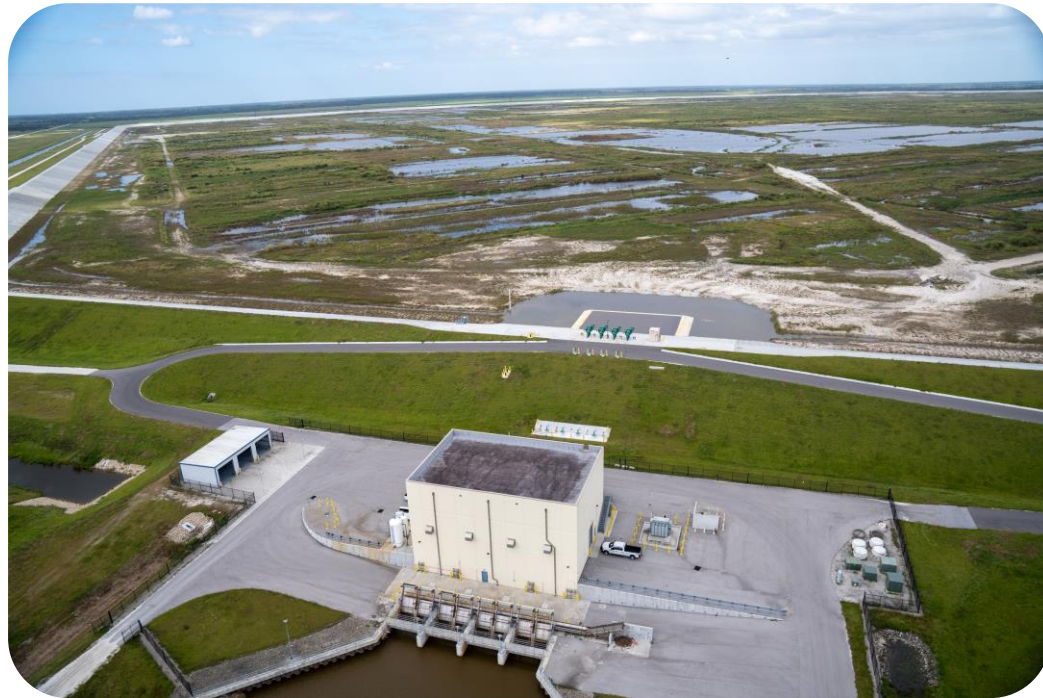
C-44 Reservoir and S-401 Pump Station
