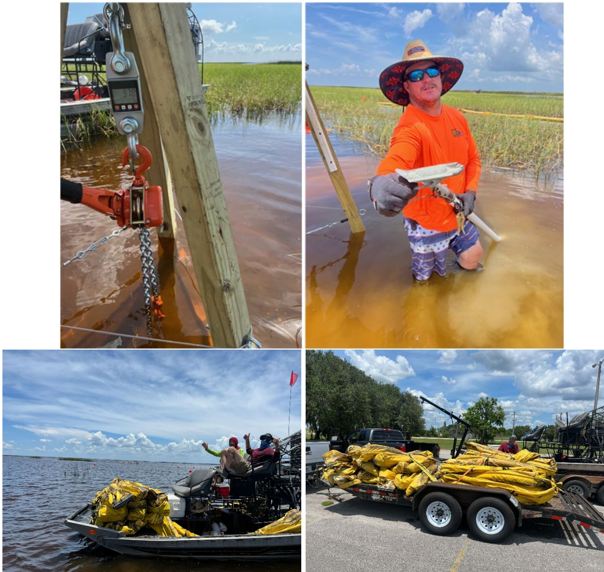
Figure 14. Anchor removal using engine hoist and tripod. Scale confirmed anchor holding power during anchor testing, installation and removal.
