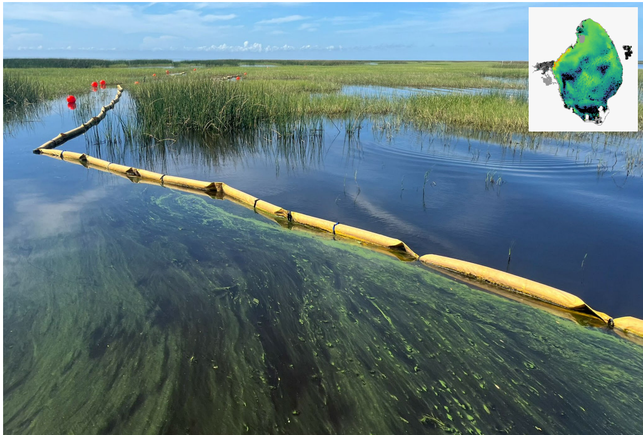
Figure 3. Turbidity controls prevented the movement of surface films and algae blooms from drifting into the area protected by the installation, shown here at the South Site on August 6, 2025. Inset shows the Cyanobacteria algal bloom monitoring image for the same date, with higher cell densities in red along the Indian Prairie shoreline where the project was located. Image derived from Copernicus Sentinel-3 satellite data as processed and available from NOAA Coastal Centers for Ocean Science at https://coastalscience.noaa.gov/science-areas/habs/hab-monitoring-system/cyanobacteria-algal-bloom-satellite-lake-okeechobee-fl/
