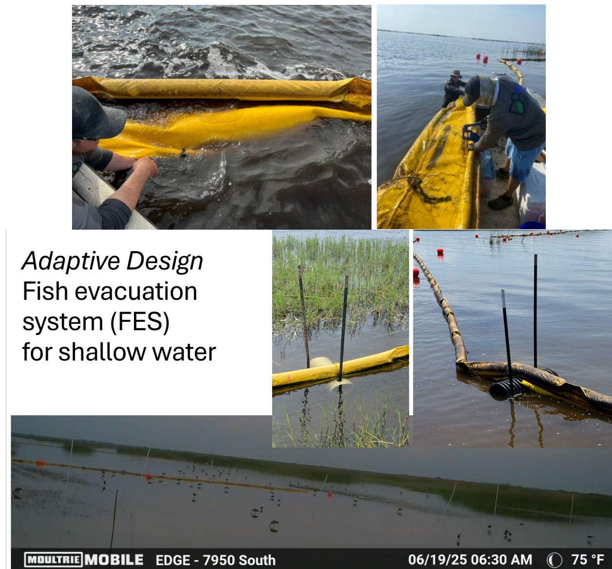
Figure 13. Installation of Fish Evacuation System to avoid entrapment of fish in shallow water when lake levels recede.
