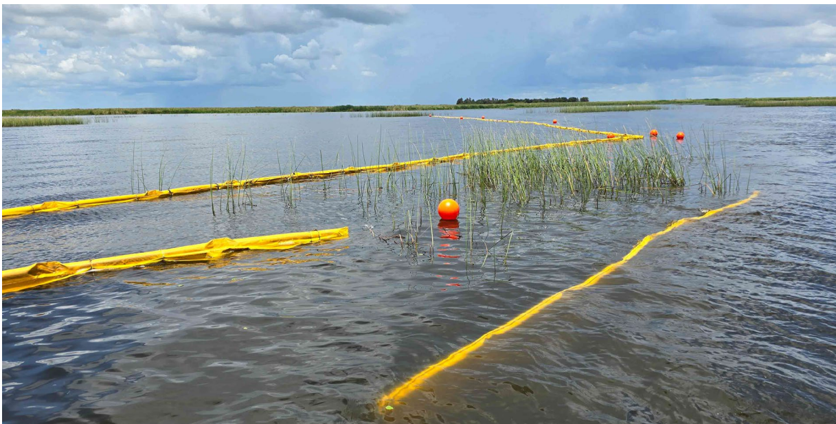
Figure 1. Turbidity controls deployed in Lake Okeechobee. Silt fence in the foreground extends from the lake bed upward, preventing turbid water from moving along the lake bed, but allowing surface water to pass over the fence during storms. The overlapping boom and barriers (“curtains”) in the background float at the water surface and are effective at redirecting surface films and surface water flows, but leave a gap between the bottom of the curtain barrier and the lake bed for water and wildlife to pass through.
